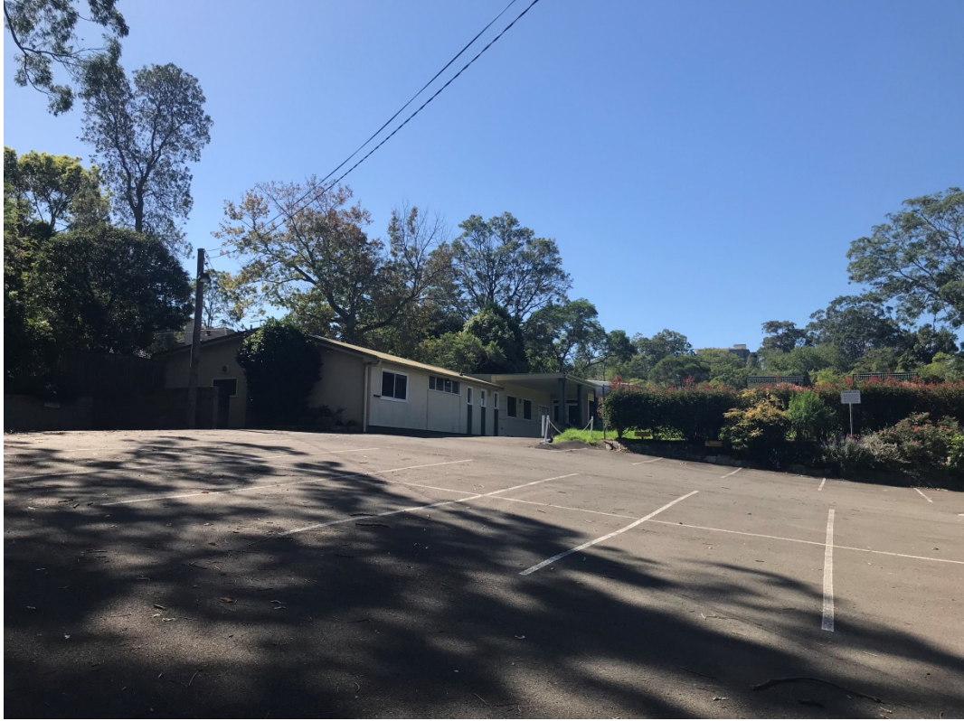
Carpark and clubhouse (Lot Y DP387680) - 4 Pennant Avenue, Gordon
