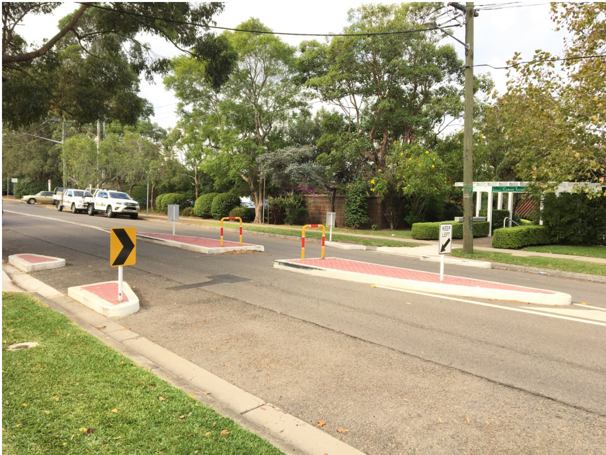
Pedestrian Refuge Island, Cowan Road St Ives
