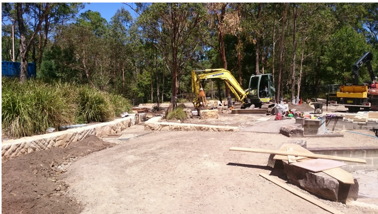
Construction of Bicentennial Park Golden Grove Playground, West Pymble
