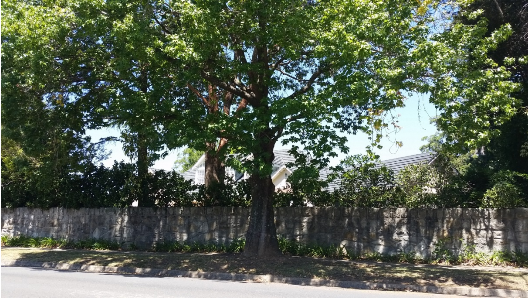
Image 1: Example of sandstone fences along Telegraph Road
