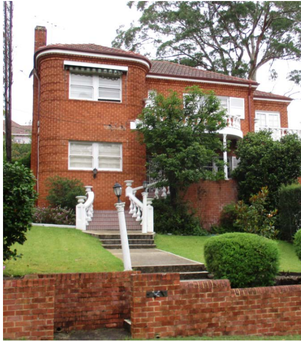
Image 1: 9 Kywong Avenue retains its original face brick façade and original windows; modifications include replacement balustrades
