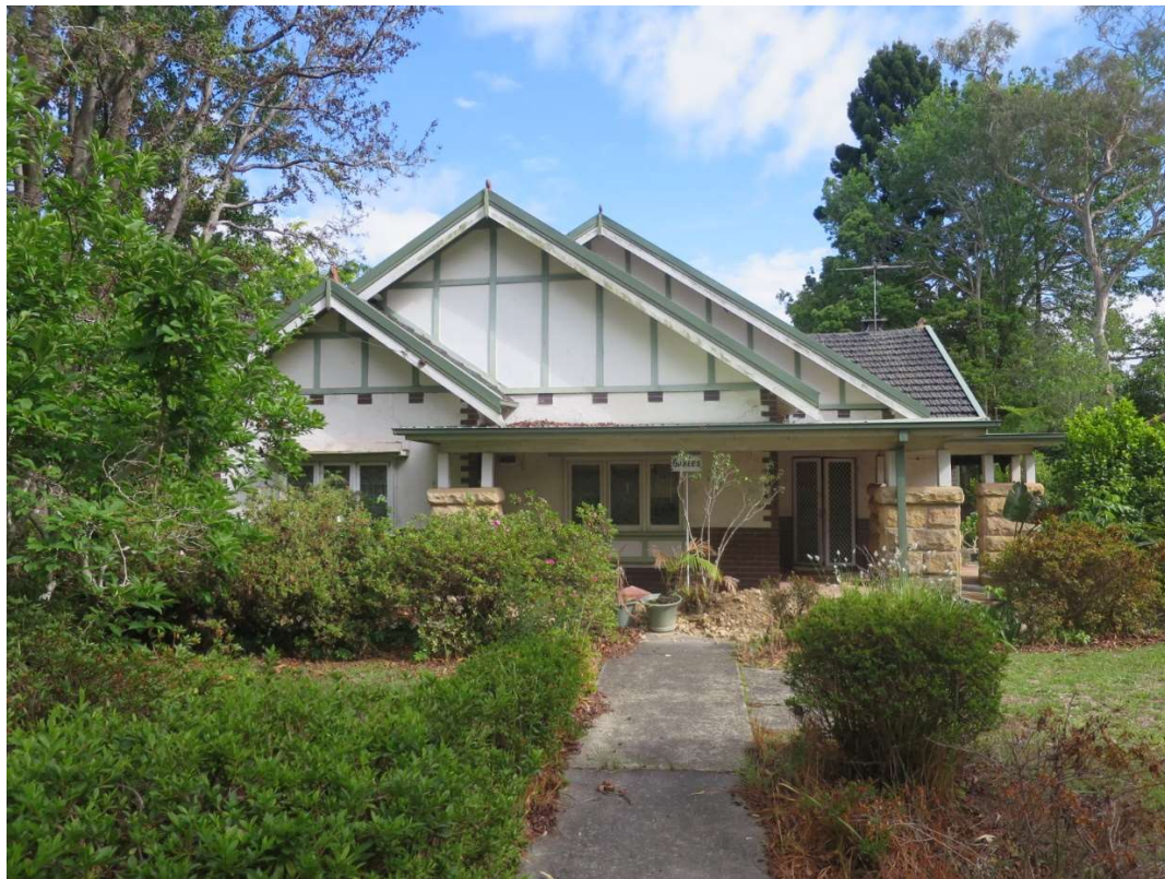
Figure 2 - Primary facade as viewed from Kissing Point Road.
