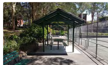
Figure 10 - Existing shelter area setting
