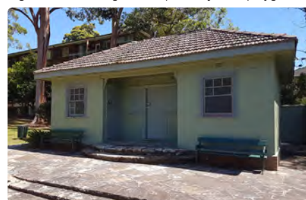
Figure 05 - Existing Tennis Pavilion
