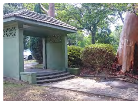
Figure 07 - Existing Gateway Pavilion
