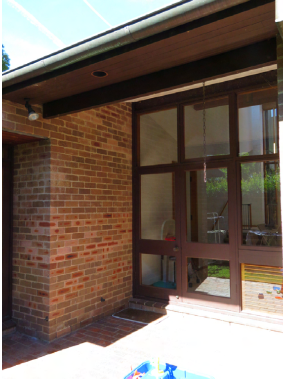
Figure 6: Family Room on the north-east side with the doors and window deeply recessed to shade them from the sun (Photo: Robertson & Hindmarsh Pty Ltd, March 2020)
