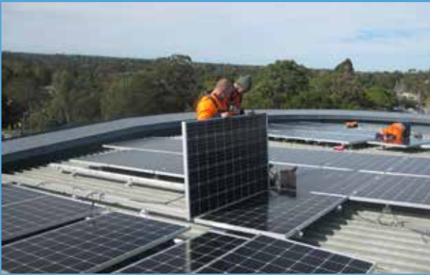
Solar PV panels being installed
