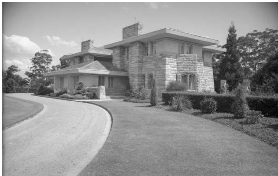
Figure 4 — View of the house from the entry on the corner of Telegraph Road showing the curvilinear driveway and the formal garden on the right.
