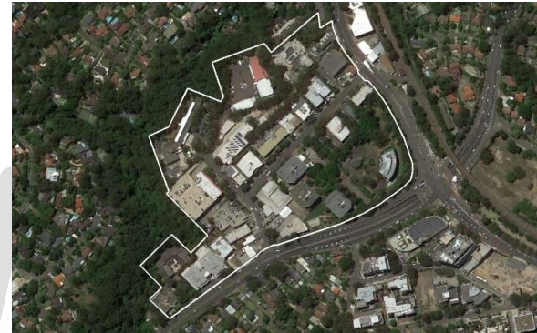
Figure 4.6 Satellite View of Pymble Business Park
