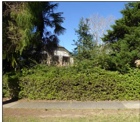
FIGURE 24: 10 LORNE AVE, VIEW FROM STREET. HERITAGE ITEM BARELY VISIBLE BEHIND TREE AND SHRUBBERY SCREENING. (SOURCE: CURIO 2016)
