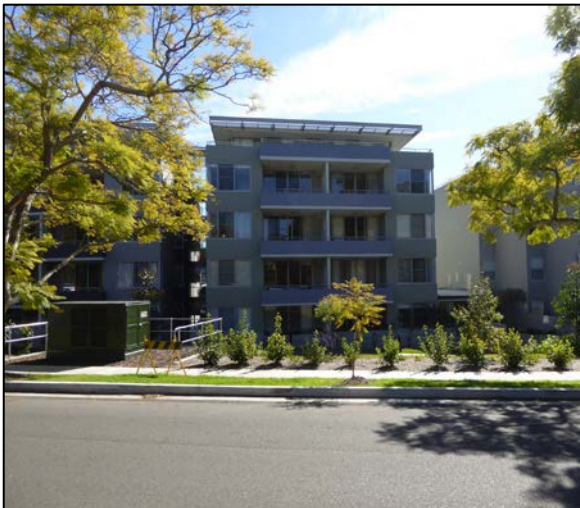
FIGURE 26: MATURE TREES AND YOUNG PLANTINGS IN FRONT OF 3-7 LORNE AVENUE APARTMENTS. (SOURCE: CURIO 2016)
