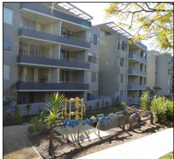
FIGURE 17: 3-7 LORNE AVENUE, NEW APARTMENT COMPLEX (SOURCE: CURIO 2016)
