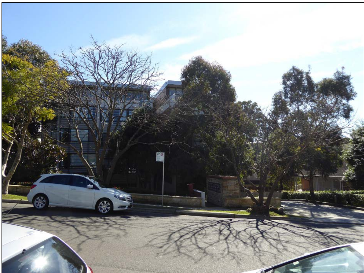
FIGURE 20: 29 LORNE AVE APARTMENTS, WEST OF SUBJECT SITE. (SOURCE: CURIO 2016)
