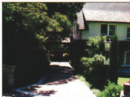
Figure 2.39 View of the western façade of the building and carport.
