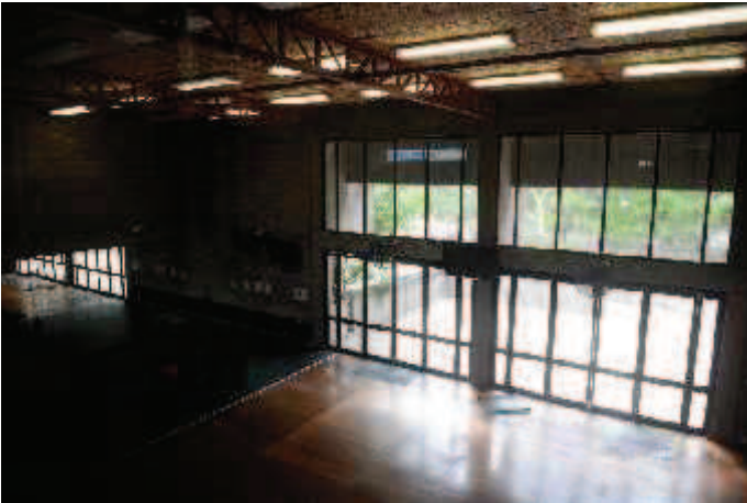
PERFORMANCE SPACE - FLOOR, STRAWBOARD CEILING, LIGHTS & DAMAGED METAL LOUVRES
