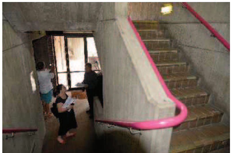
GYMNASIUM - STAIR HANDRAILS
