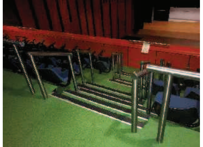
AUDITORIUM – LOW HEIGHT BALUSTRADE, HANDRAILS
