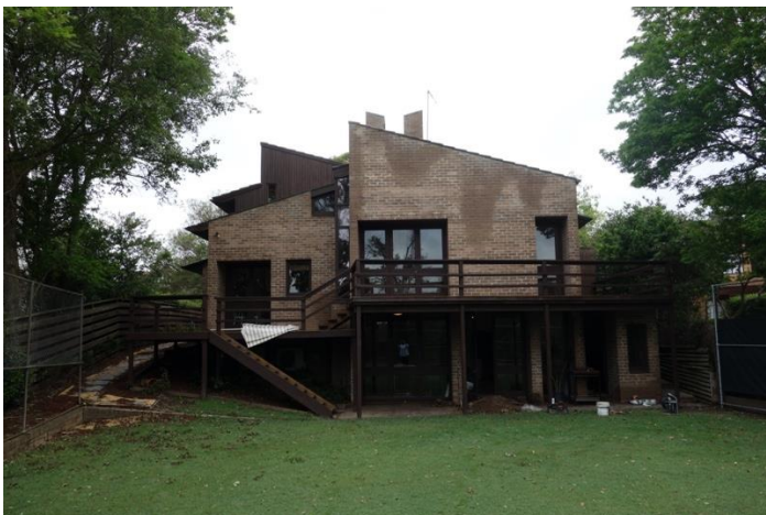
View to the rear elevation of the subject building.
